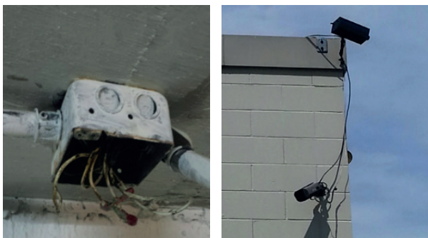
Some example of improper installation of CCTV on premises
